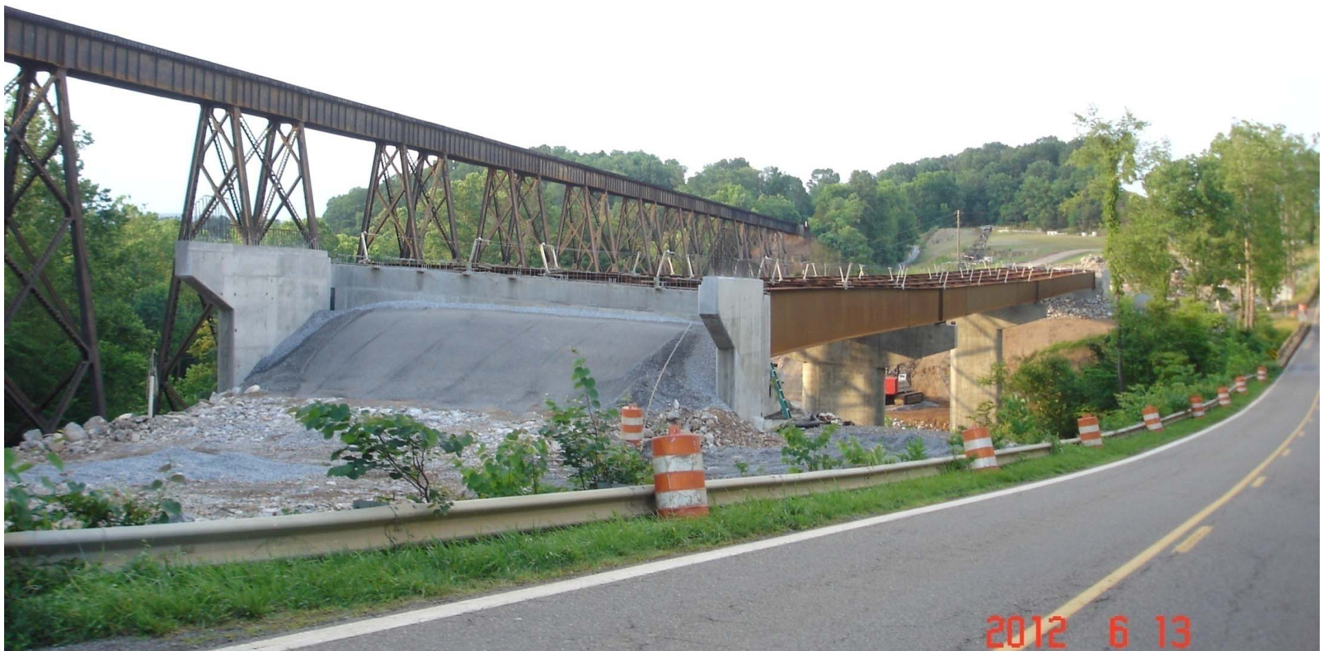
View from Abutment A – looking north.
