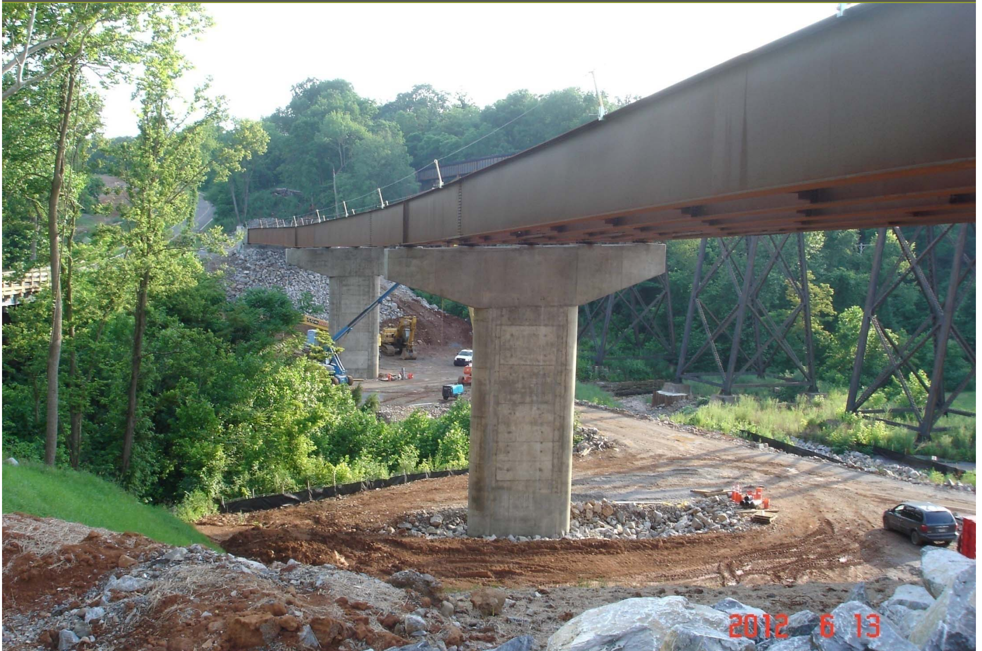
View south, Pier 2, with Pier 1 in background.
